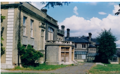
Pictures: (Top Left) Roof repair c1980 (Bottom) Georgian and North Wings 1993 (Top Right 1-3) Georgian Wing 1993 (2) / Eastern Elevation 1993
